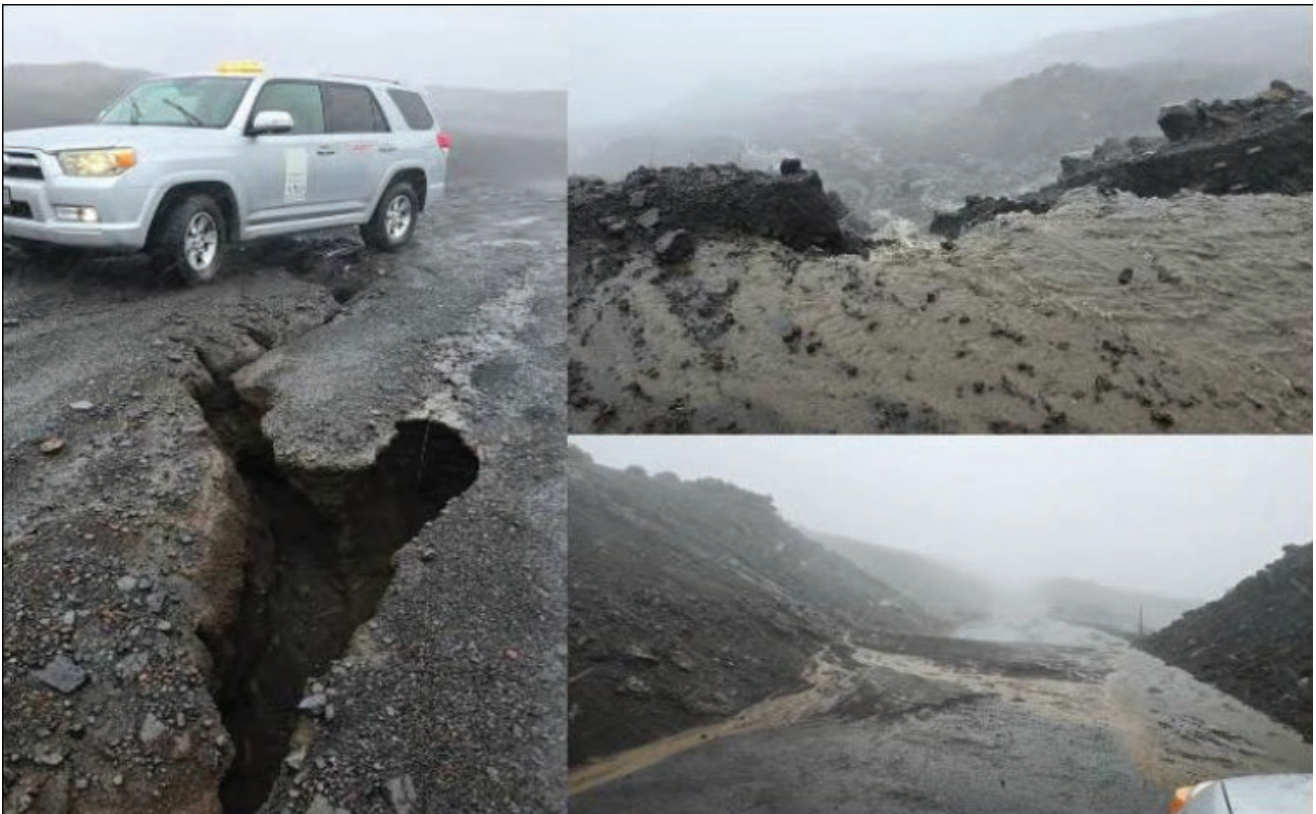
Figure 9. Hurricane Hone Damage.
