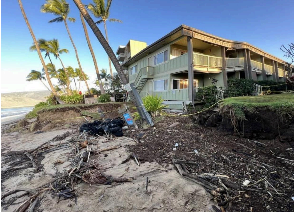
Figure: Housing damaged by 1/25 flood, likely this will be condemned.
