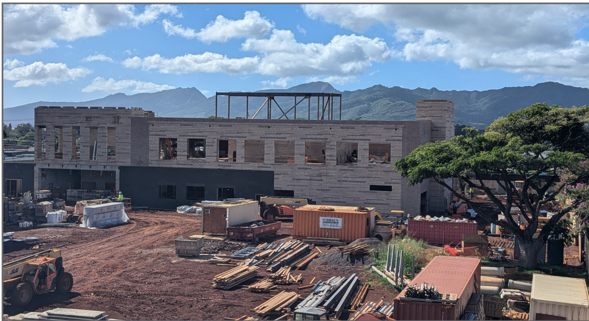
Vertical concrete walls of the new Wahiawā Civic Center's two-story structure rise above the construction barrier that surrounds the site, December 11, 2024.
