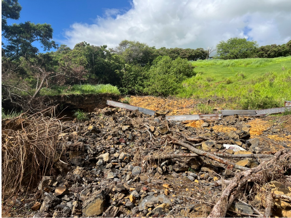
Photo 15- Blown Out Levee Above MP 60 (Looking Northwest)
