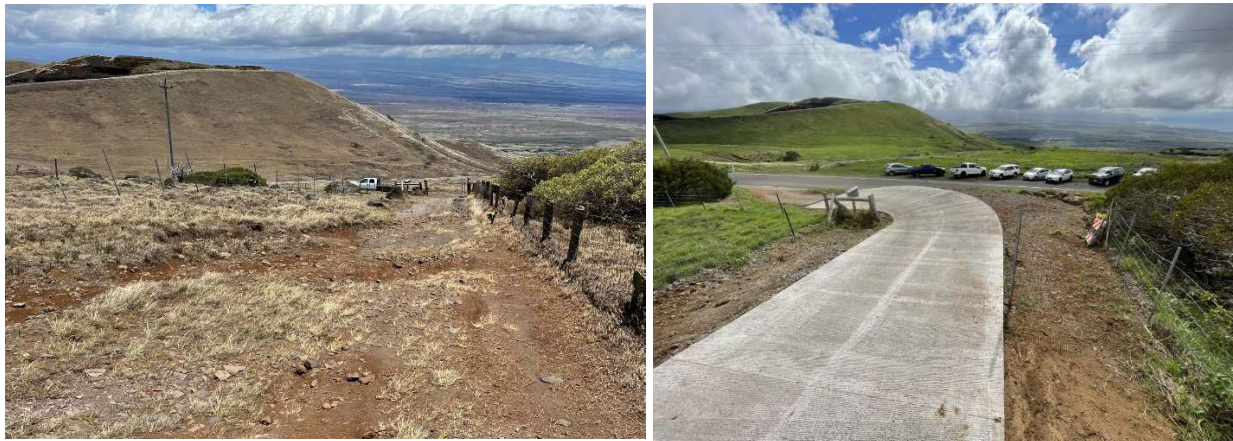
Before and after images of the Koai‘a Corridor access improvement project.
