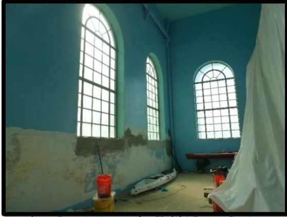
Repainting at the Kalihi Pump Station
