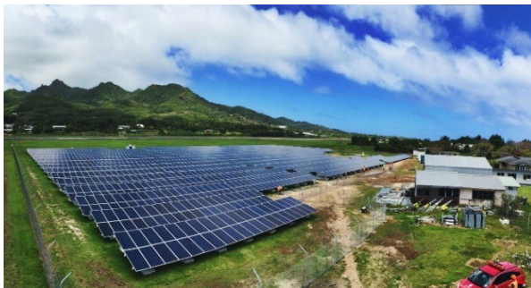
Figure 2. Te Mana o Te Ra PV + BESS project (1 MW, 5.6 MWh) at the Rarotonga International Airport.
