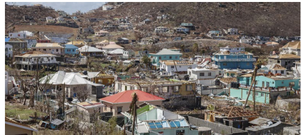
Figure 2. Homes destroyed by Hurricane Beryl in 2024.
