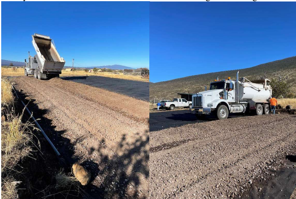
Photo 4 and 5. Delivery and spreading of aggregate material to prepare additional sites to support the East Hawaii Wildlife game program. East Hawaii
