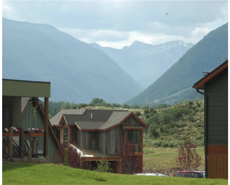
Burlingame Range, Phase I, Aspen, CO Image Source: Aspen/Pitkin Co. Housing Authority
