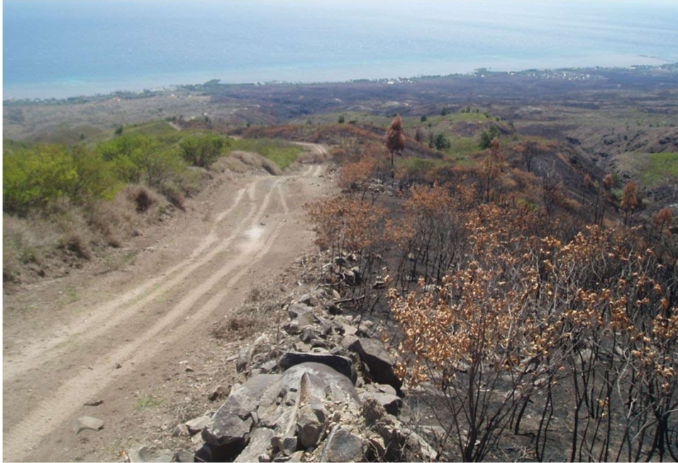
A firebreak road installed by the East Molokai Watershed Partnership prevented a fire from spreading east (left) in 2009. A similar fire that burned before the firebreak spread twice as far a decade earlier.
