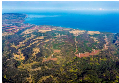
Kawailoa Wind Power, O'ahu
