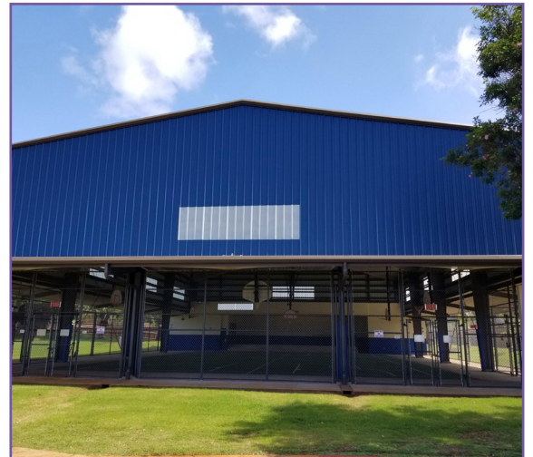
The Waimea Canyon Middle School Covered Play Court is finally completed
