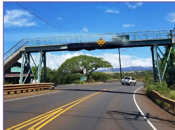
'Ele'ele Pedestrian Bridge.
