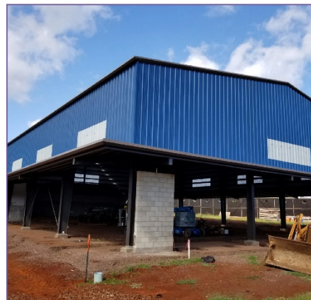
The Waimea Canyon Middle School covered play-court is nearing completion.
