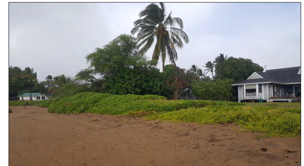
Photo: A vegetated sand berm protects a house from waves and flooding.
