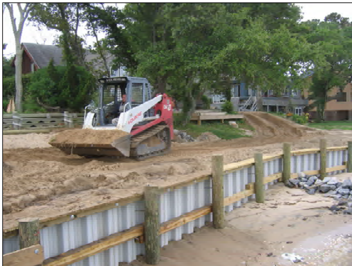
Photos: A typical vinyl and wood pile bulkhead.
