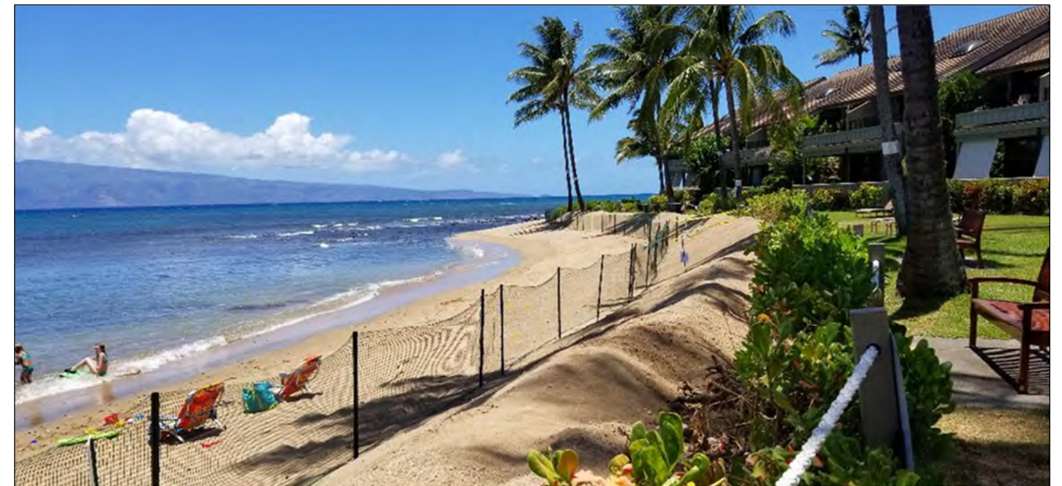
Photo: Sandy berm with a sand-filled coir burrito before planting at Kahana Bay, Maui, HI.
