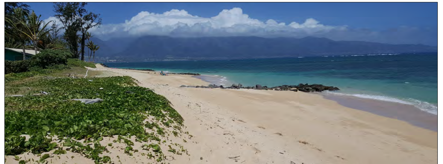
Photo: A series of short rock groins have retained the beach at Stables Road, Maui.
