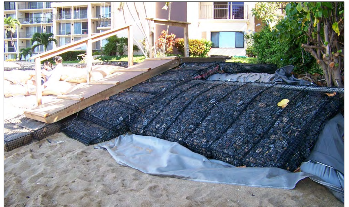
Photo: Tensar brand rock filled mattress underlain by geotextile fabric.
