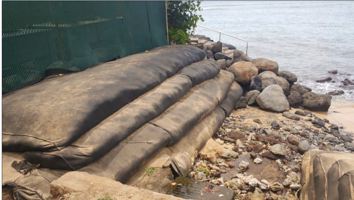
Photo: A stack of sand-filled burritos made of black Mirafi filter fabric, West Maui, 2018.
