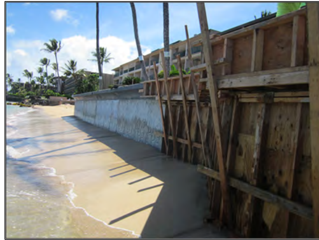
Photo: A poured concrete seawall.
