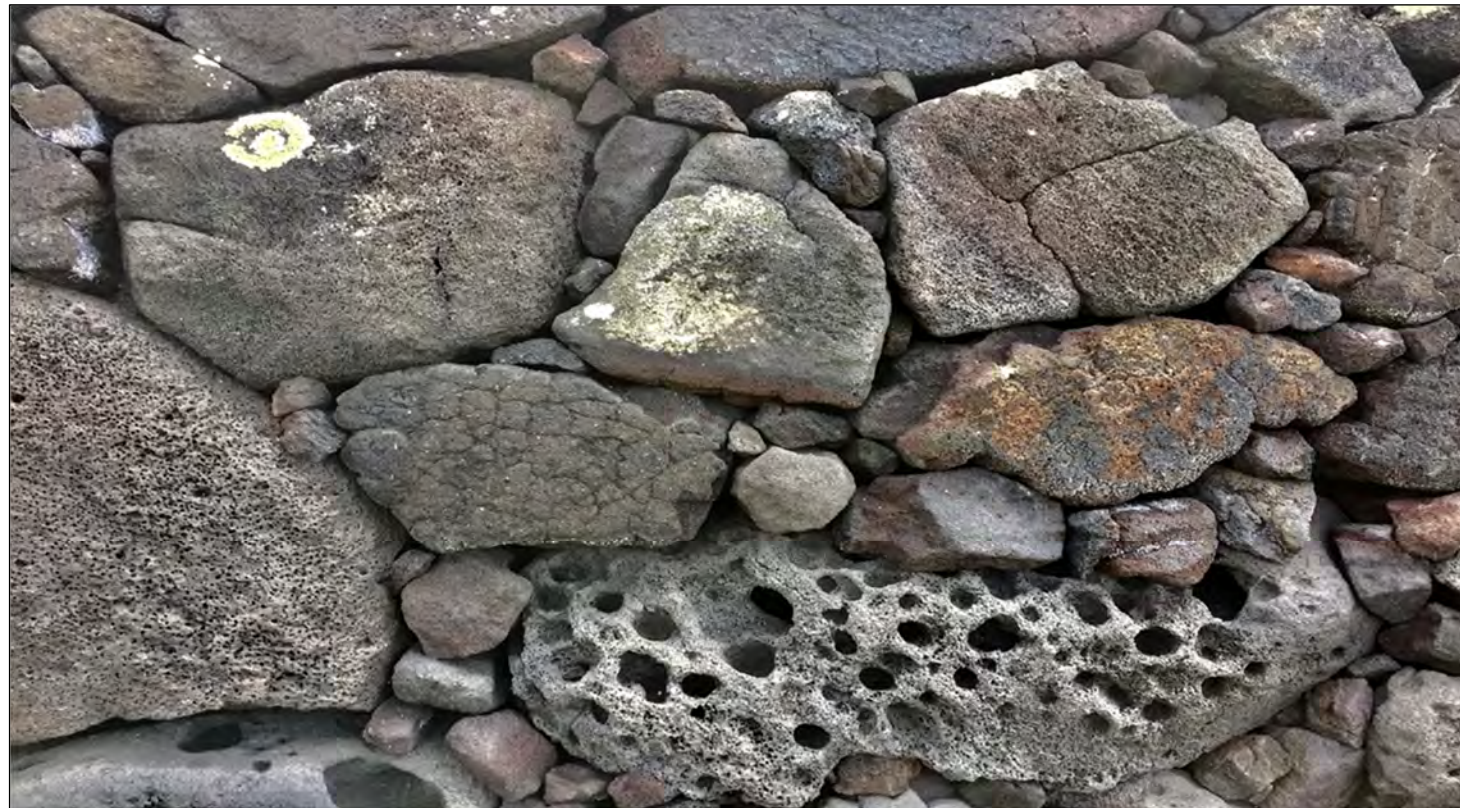
Photo: The intricate structure of a wall constructed using u hau humu pōhaku (Hawaiian dry-stacked masonry). Source: National Park Service Photo. https://www.nps.gov/puho/learn/historyculture/preservation.htm
