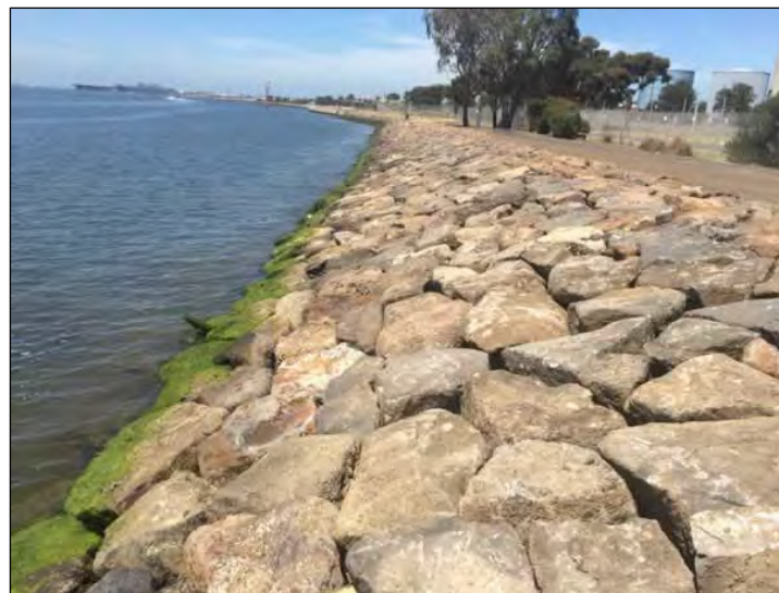
Photos: A properly designed revetment has interlocking stones underlain with geofabric.
