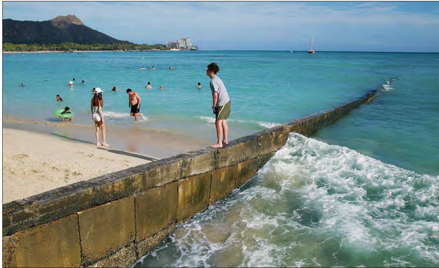
Photo: A concrete block groin illustrates updrift accretion and down drift erosion at Kūhiō Beach, Waikiki, Oahu, Hawai'i.
