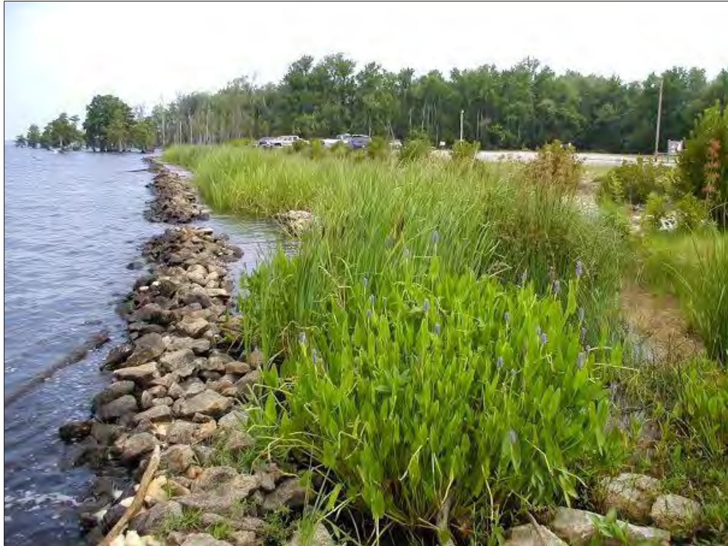
Photo: An example of a vegetated sill. Source: North Carolina Coastal Federation. https://www.publicradioeast.org/post/living-shorelines .
