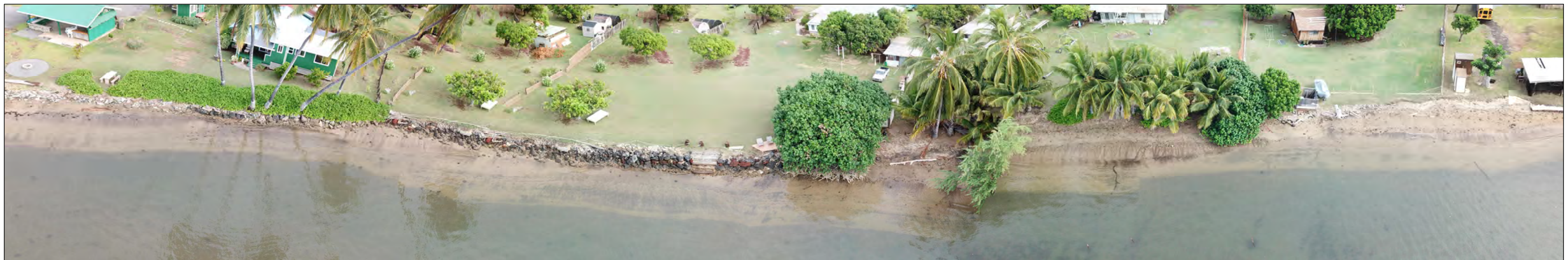
Photos (Clockwise from Top): 1. Looking east along an eroding shoreline fronting Kamiloloa; 2. Informal, shoreline armoring fronting Kamiloloa; 3. Panorama view of informal shoreline armoring and the use of naupaka along Kamiloloa (Source: DHHL).
