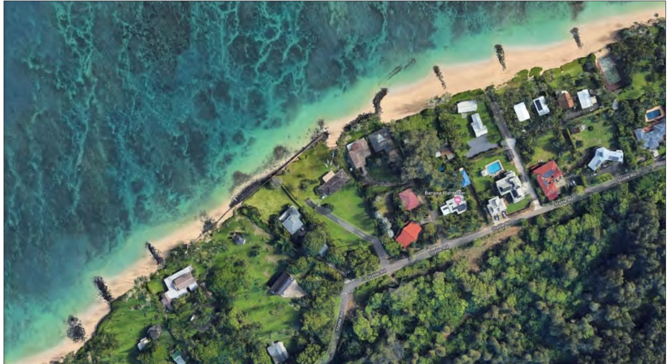
Photo: Aerial imagery of rock stub groins along Maui's north shore.
