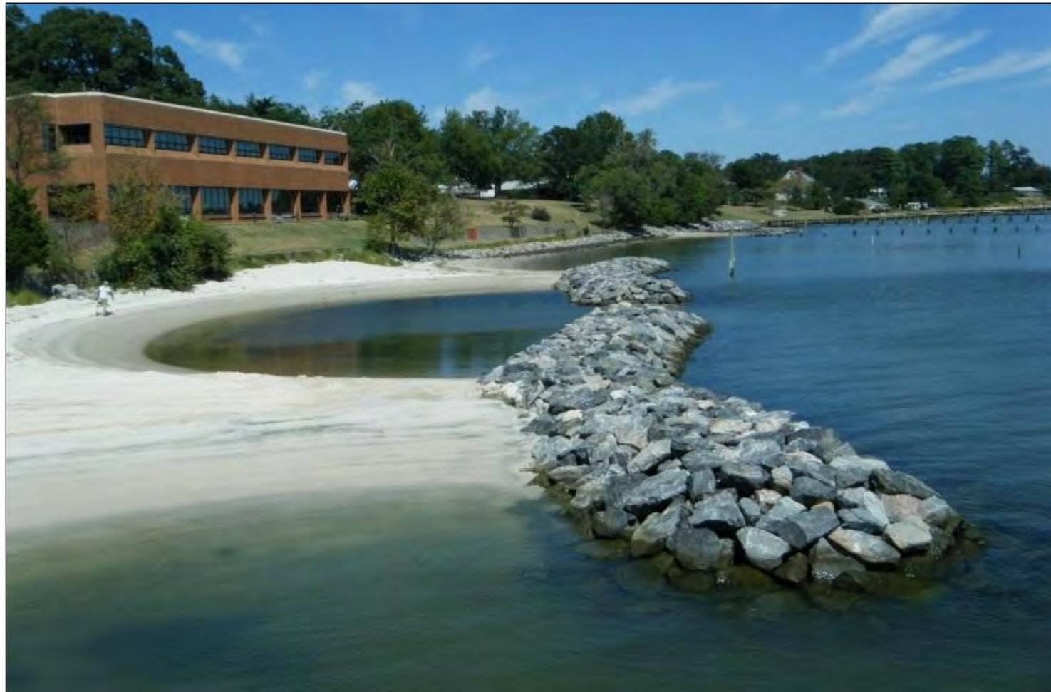
Photo: A rubble mound breakwater has accumulated sand in the eddy behind the structure. Photo by K. Duhring. Source: Center for Coastal Resources Management, Virginia Institute of Marine Science.
