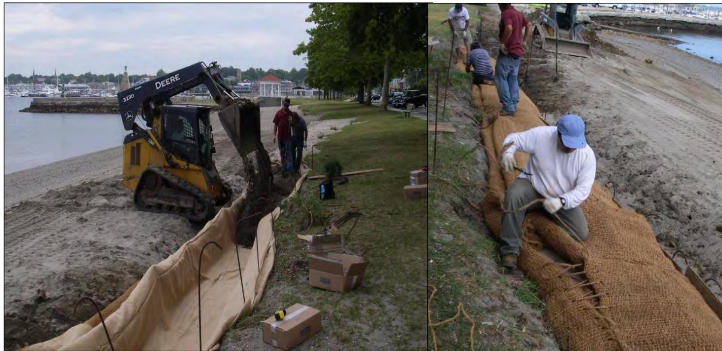
Photos: Examples of a sand-filled coir 'burrito' at King's Park, Newport, RI Photos courtesy of Janet Freedman (TNC, 2017).
