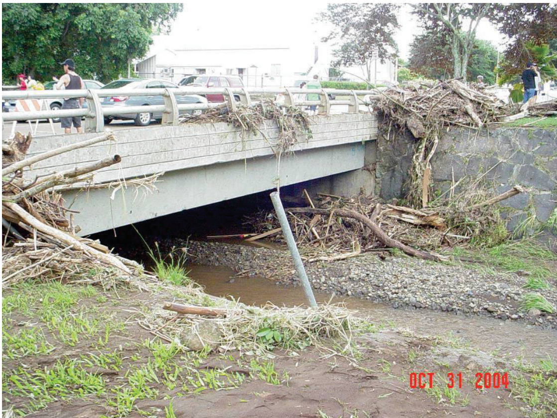
Figure 4: Debris, composed mostly of albizia, left over from the 2004 flood event in Mānoa.
