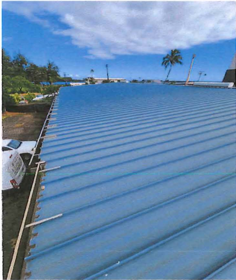
Image 1: Existing 8000sqft Roof
