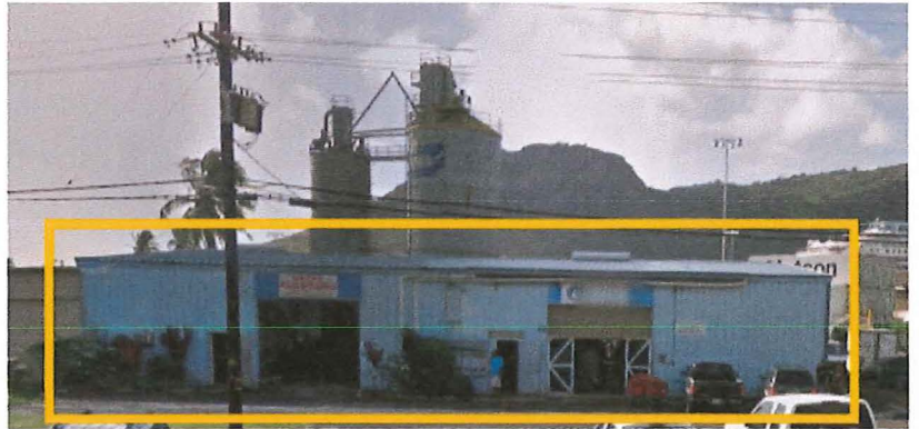
Image 2: 1650sqft Existing Siding to be replaced
