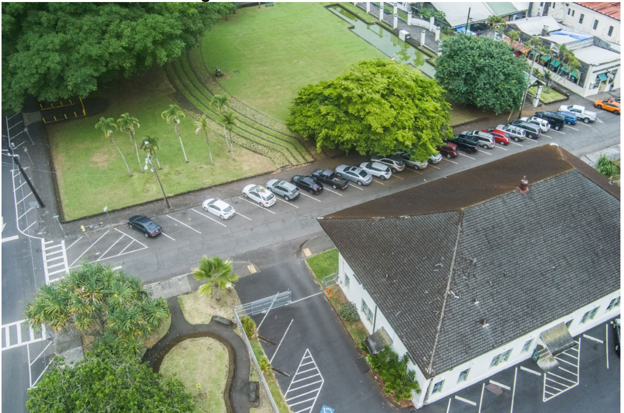
View of EHCC's roof and Kalakua Park directly across the street.
