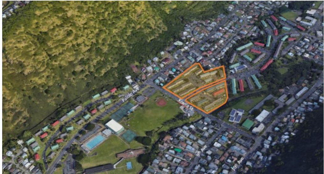
Aerial view of Palolo Valley Homes property
