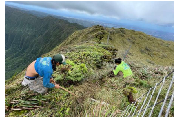
Above: Partners constructing fence in Waiawa, O'ahu. Ko'olau Mountains Watershed Partnership.
