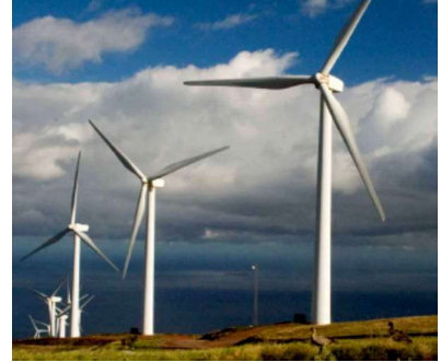
Kaheawa Wind Power project in West Maui above Ma'alaea.
