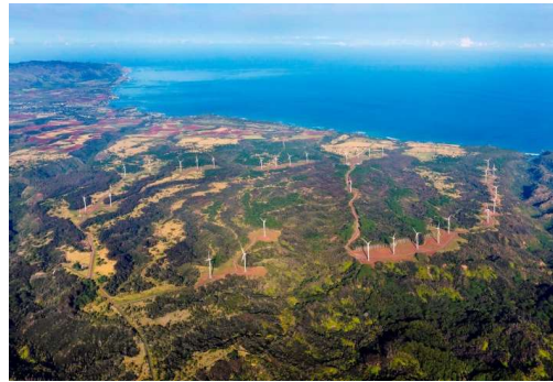
Kawailoa Wind Power, O'ahu
