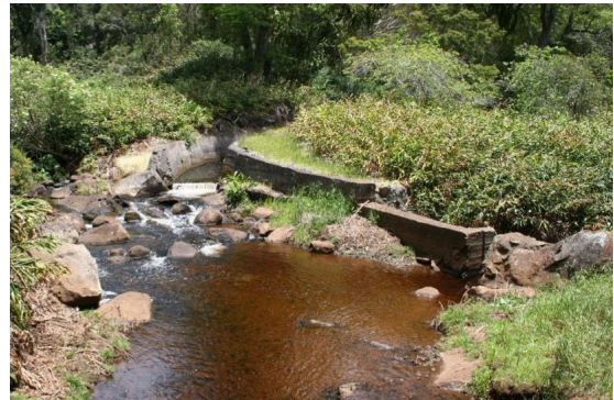
D) Diversion dam at Kōke'e Stream.
