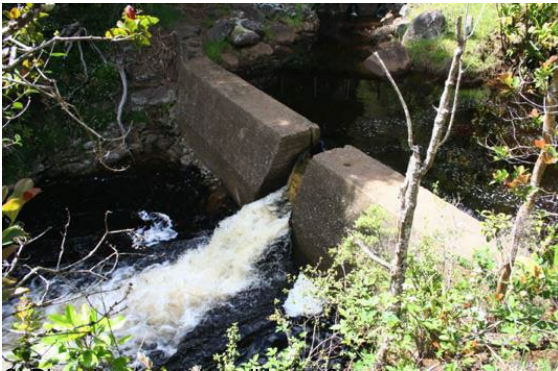
C) Diversion dam at Kauaikinana Stream.
