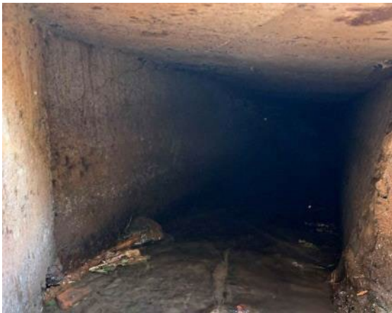
C) Water flows in an underground concrete-lined channel behind Wailuku Public Library.
