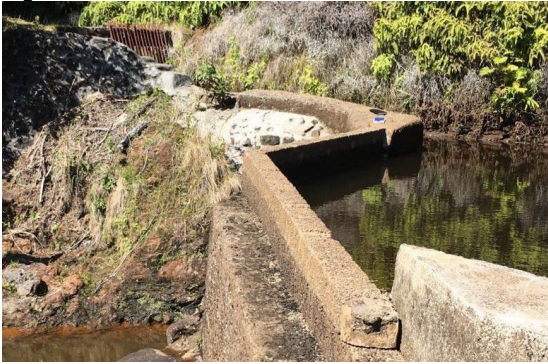
A) Diversion dam at Waiakoali Stream.
