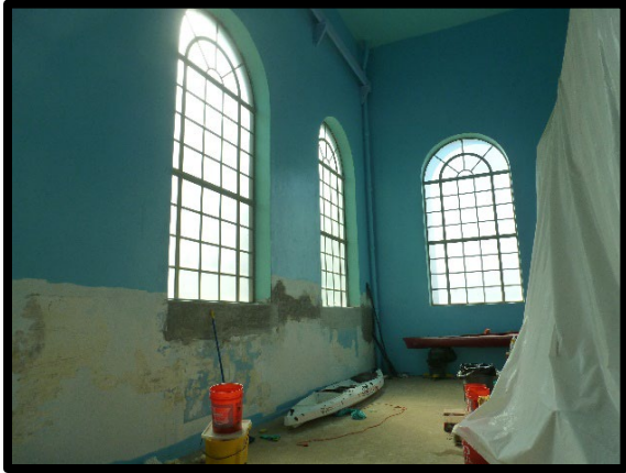
▲ Repainting at the Kalihi Pump Station
