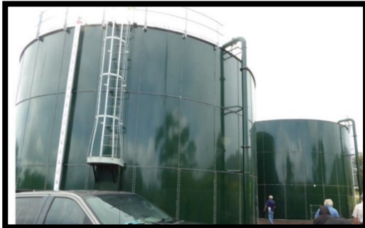
▲ New 228k-gallon steel tanks
