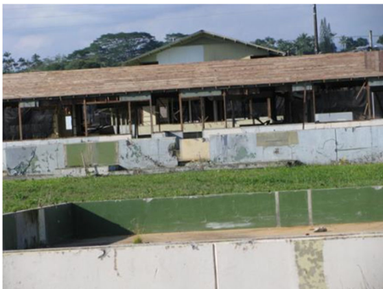
Buildings before demolition
