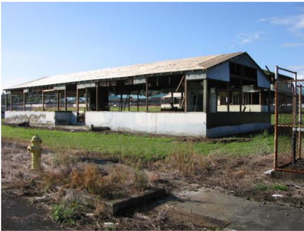
Buildings before demolition
