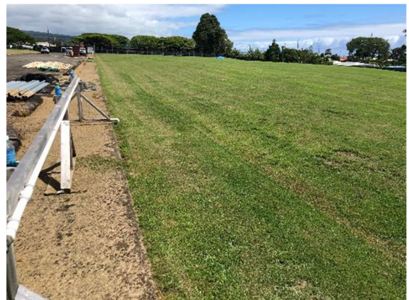
Project site after demolition and contaminated soils encapsulated
