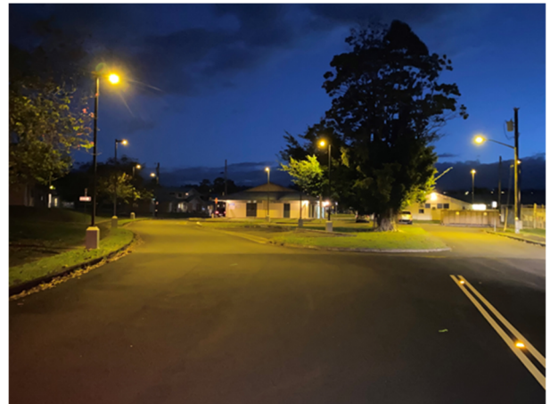
Parking lot after project completion
