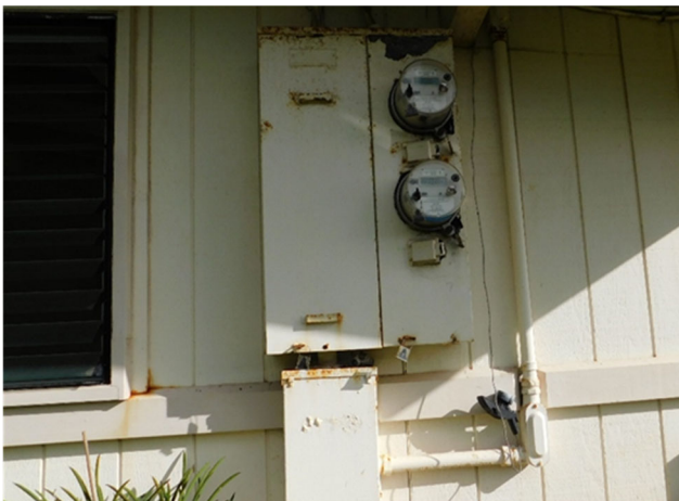
Old electrical box
