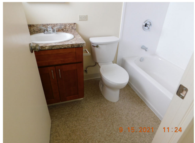
Renovated 2nd floor bathroom
