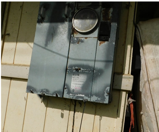
Old electrical box
