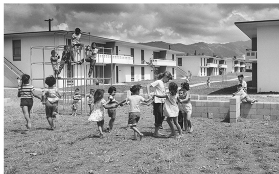
Built in 1958, the Ka'ahumanu Homes were designed to provide families ample space for outdoor living.
