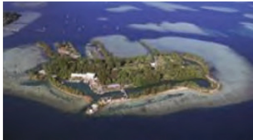
Figure 1. DC microgrid project site, Coconut Island.
