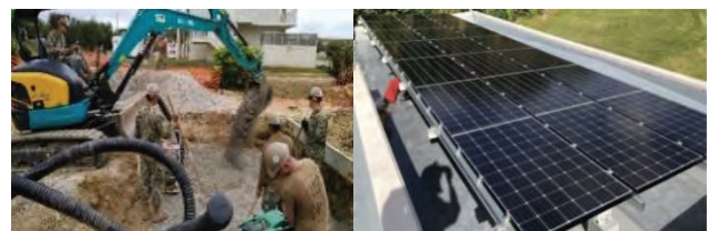
Figure 3. Project construction and new PV system.
