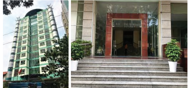
Figure 1. HCM-USTA Building, Ho Chi Minh City.
