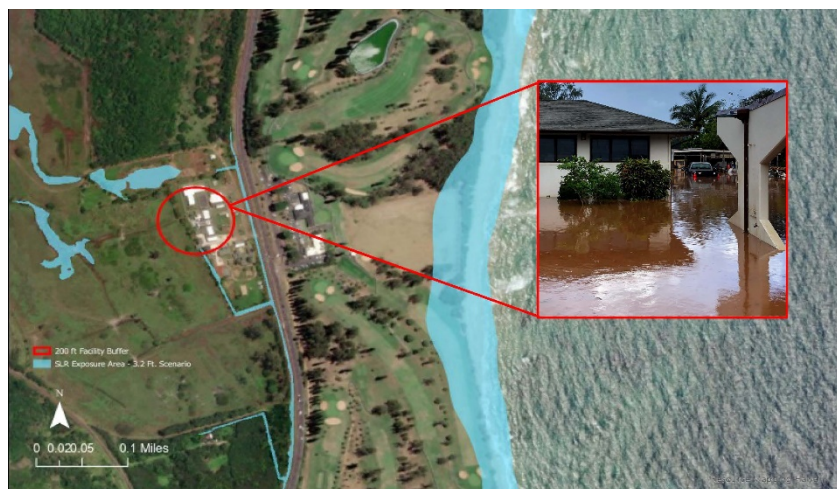
Sea level rise impacts affect not only shoreline parcels, but also low-lying areas, such as The Kauaʻi Community Correctional Center (KCCC) which experiences flooding during heavy rains. Inset photo is from a March 2020 rain event. (Photo Credit: Dept of Public Safety)
