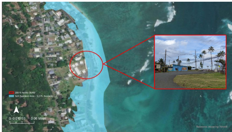
Impacts to facility access must be considered when assessing vulnerability. Ka'a'awa Elementary School, separated from the shoreline by Kamehameha Highway, is partially within the 3.2 ft SLR-XA. This projection suggests that the main building, as well as access may be impacted. (Photo Credit: OPSD-CZM)
