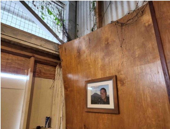
Left: vines grow in behind the plywood installed in front of the corrugated tin walls. Right: bronze gongs tarnish and corrode when protective covers are being laundered due to constant soiling by stray cats.
