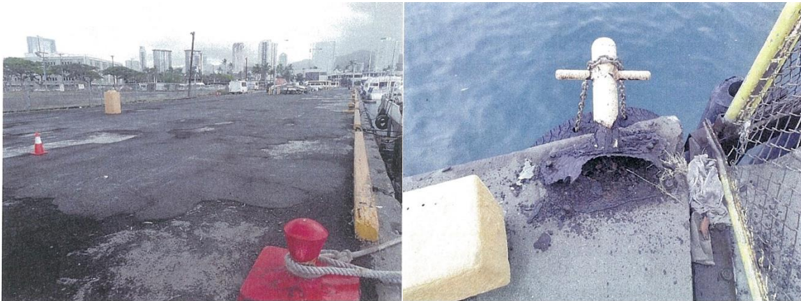
Dock surface deterioration, and mooring cleat corrosion (near collapse). Prestressed plank with broken prestressing strands in 2017 photo, extensive beam spalling and fractured beam bottom below Dock.
