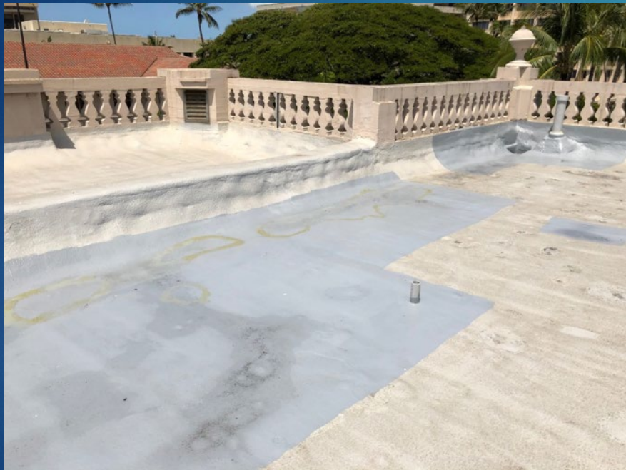
Temporary repairs along the parapet.
