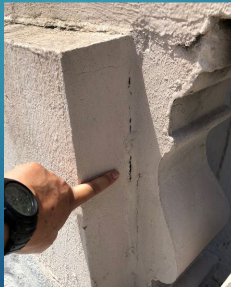
Temporary repairs along the parapet.
