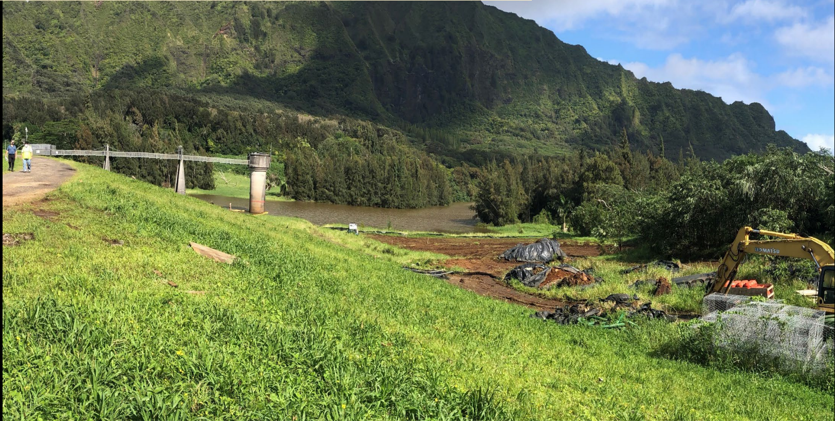
Nuuanu Dam No 4, Oahu (Improvements, Feb 2021)
