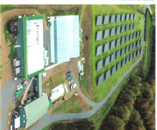
1 Megawatt Photovoltaic Farm
