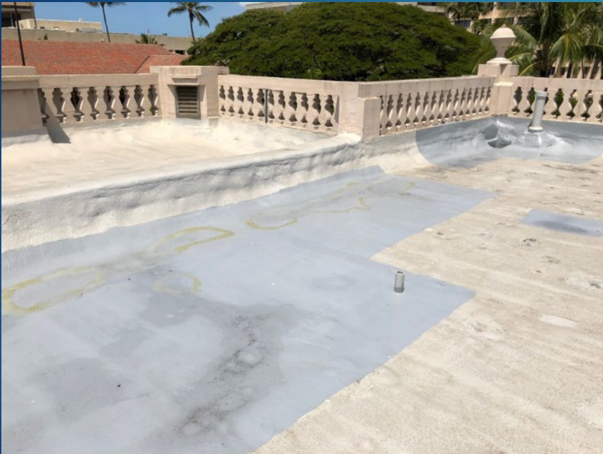
Temporary repairs along the parapet.
