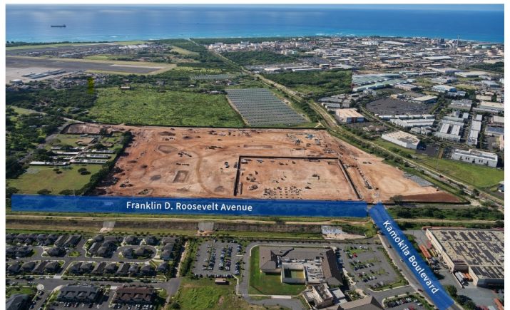
Roosevelt Ave./ Kamokila Construction, March 2022
