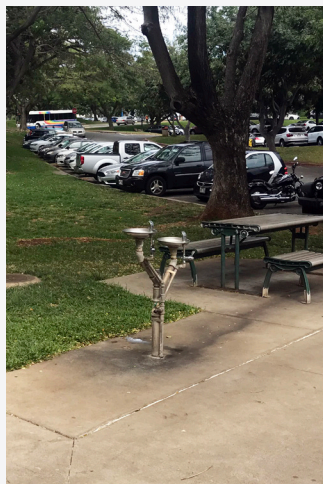
AFTER: repaired fountain
