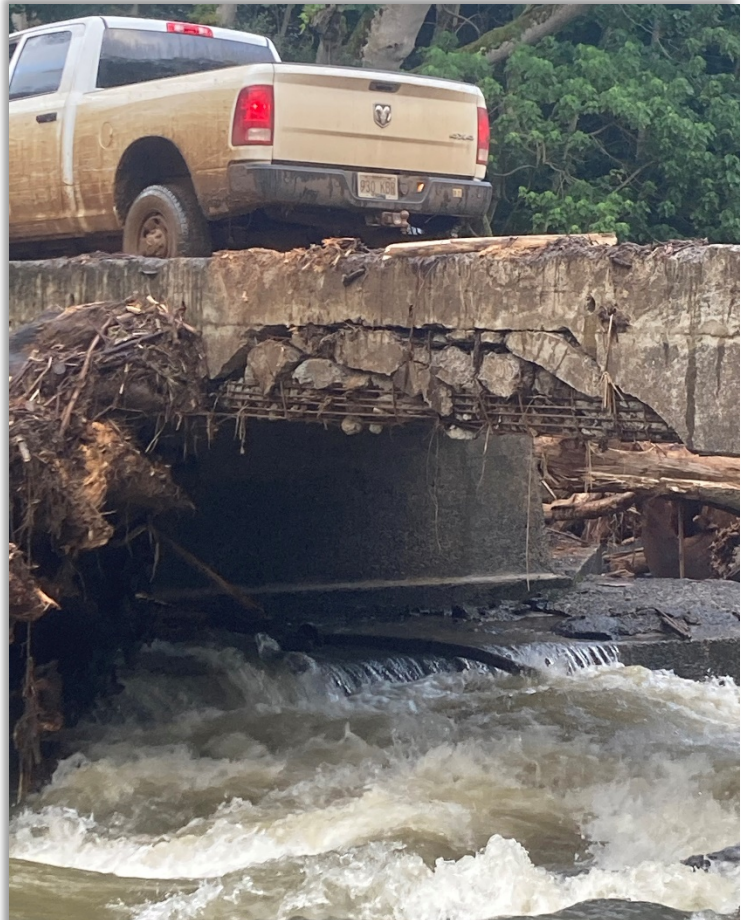
Image 1: Damage to Christian Crossing Bridge from flooding.
