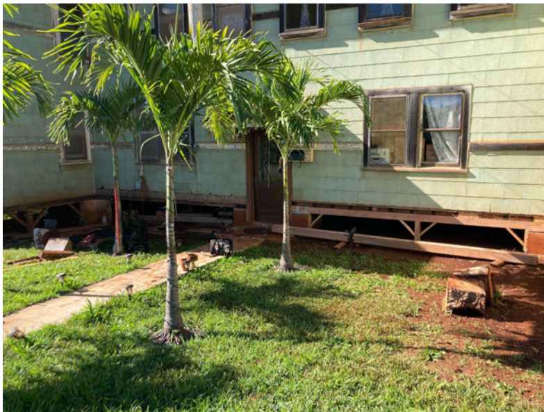
After the foundation beams were replaced
