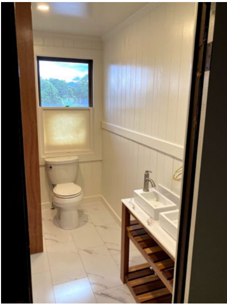
After photos of the ceiling, floor, toilet, and sinks
