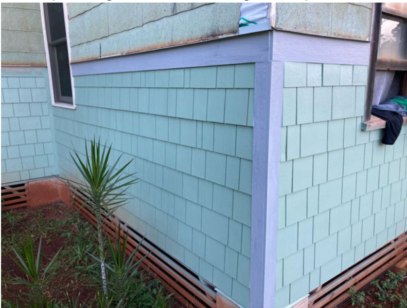
After paneling on the side of the building has been replaced
