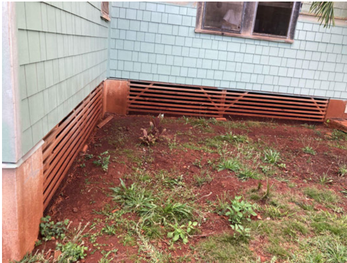
After photo foundation beams
