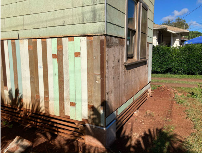
Before paneling on side of building was replaced
