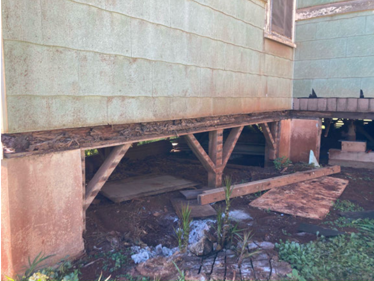
Before the foundation beams were replaced
