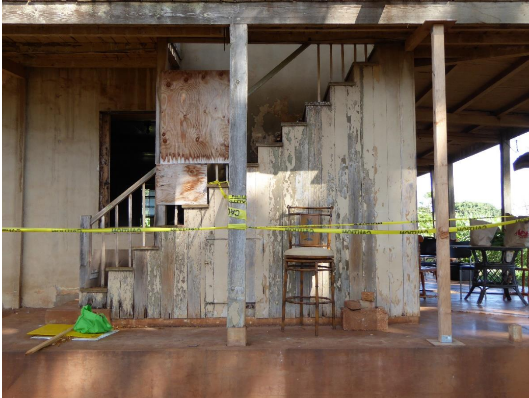
Figure 48: Exterior wood stair. Photo taken in 2015.
