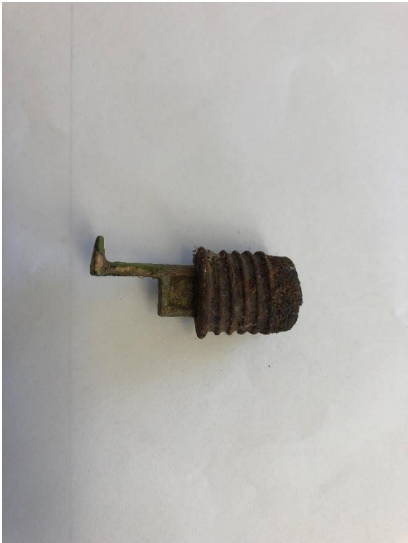
Figure 25: Typical spring sash holder used in all windows except one.
