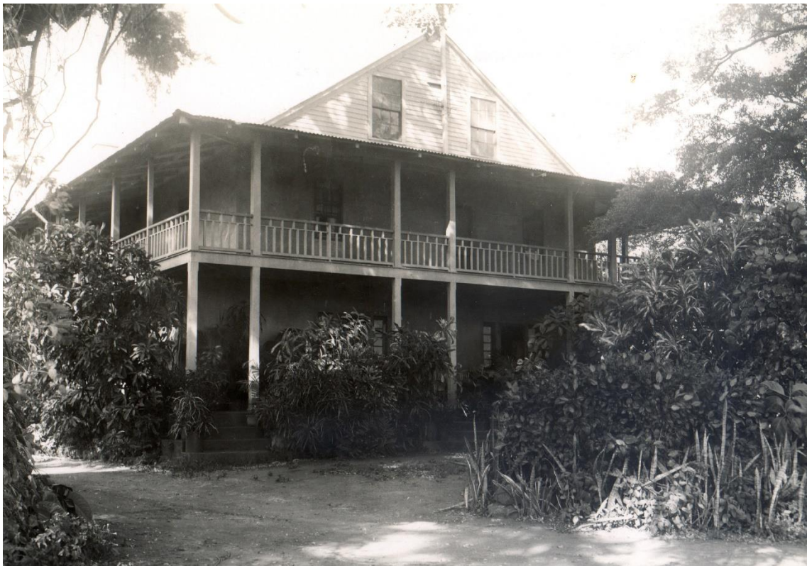
Figure 3: Photo taken in 1961 by Ray Jerome Baker. Shows change in design of railing and post locations after 1927. Note possible flagpole at south gable.
