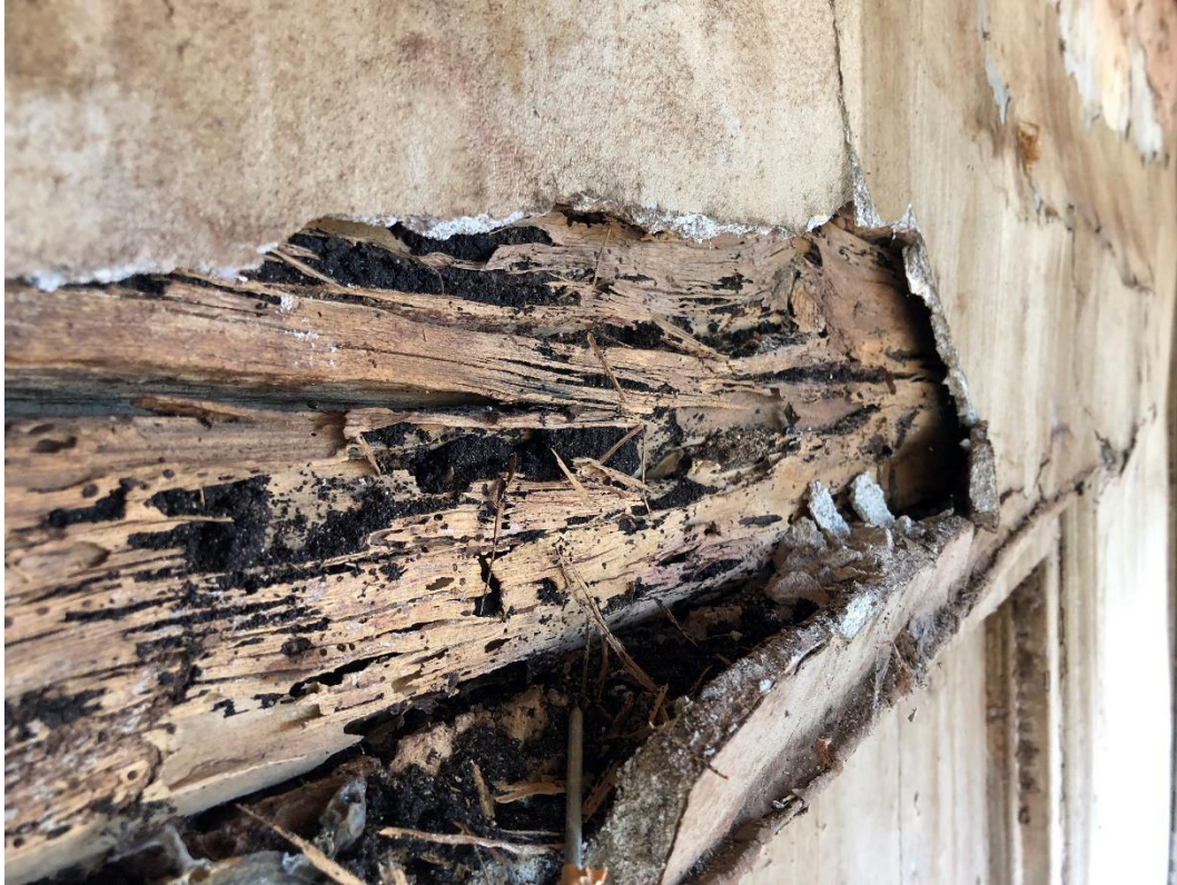
Figure 14: Lintel over window 10
