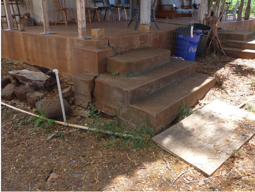
Figure 46: Stair at southwest corner
