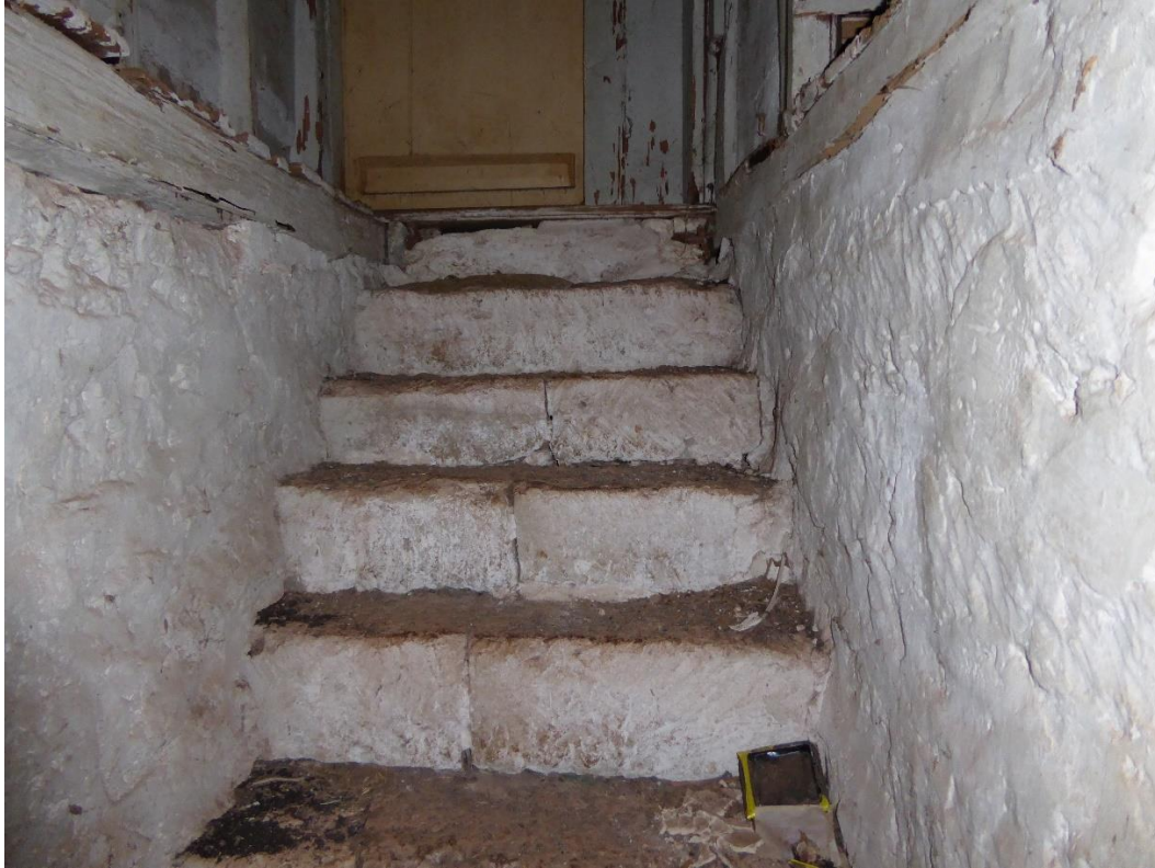
Figure 44: Stair from cellar to first floor
