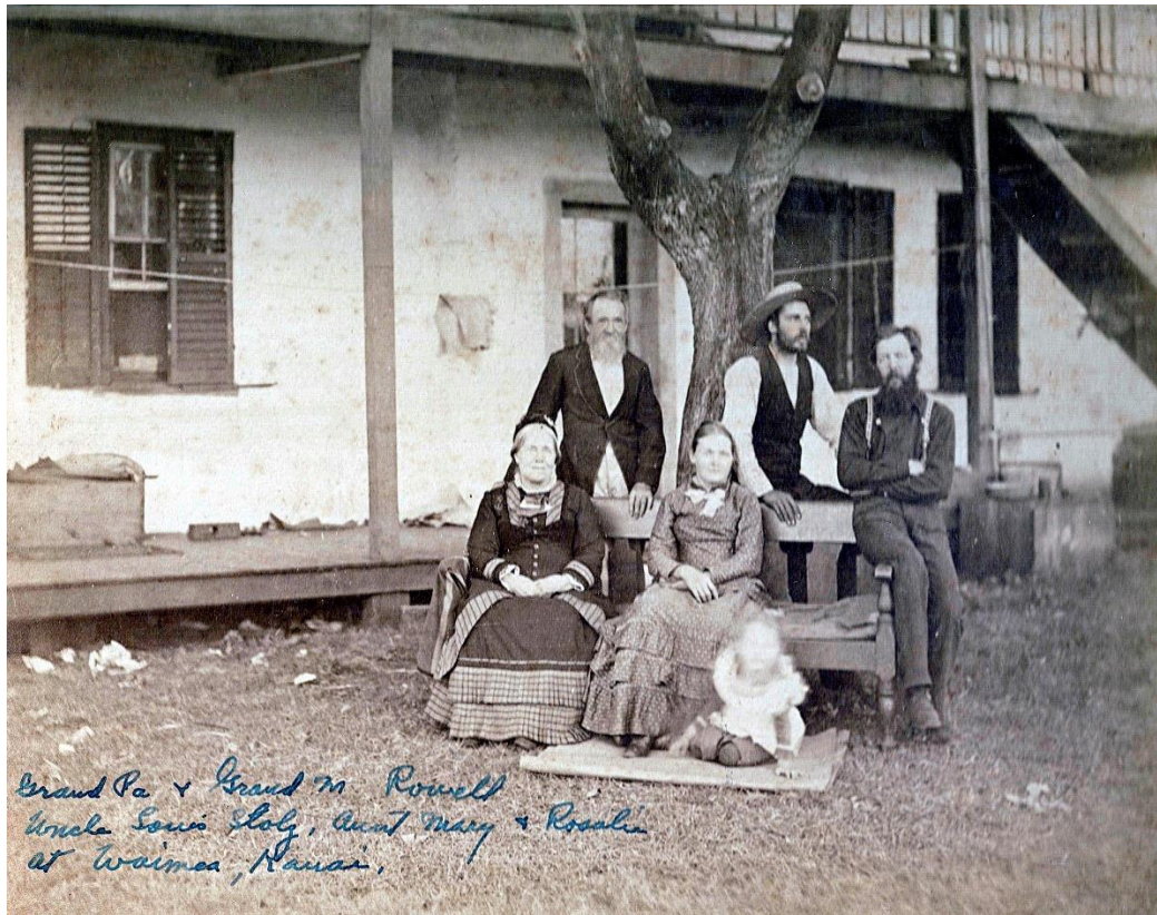
Figure 6: Original decks were wood framed.
