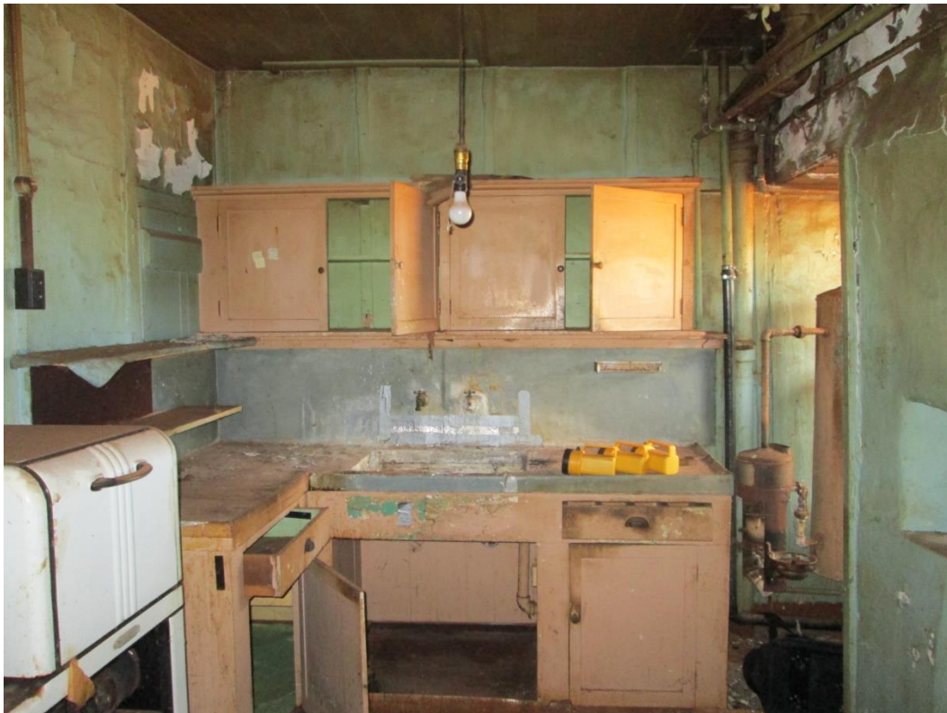
Figure 55: Kitchen sink and cabinet.
