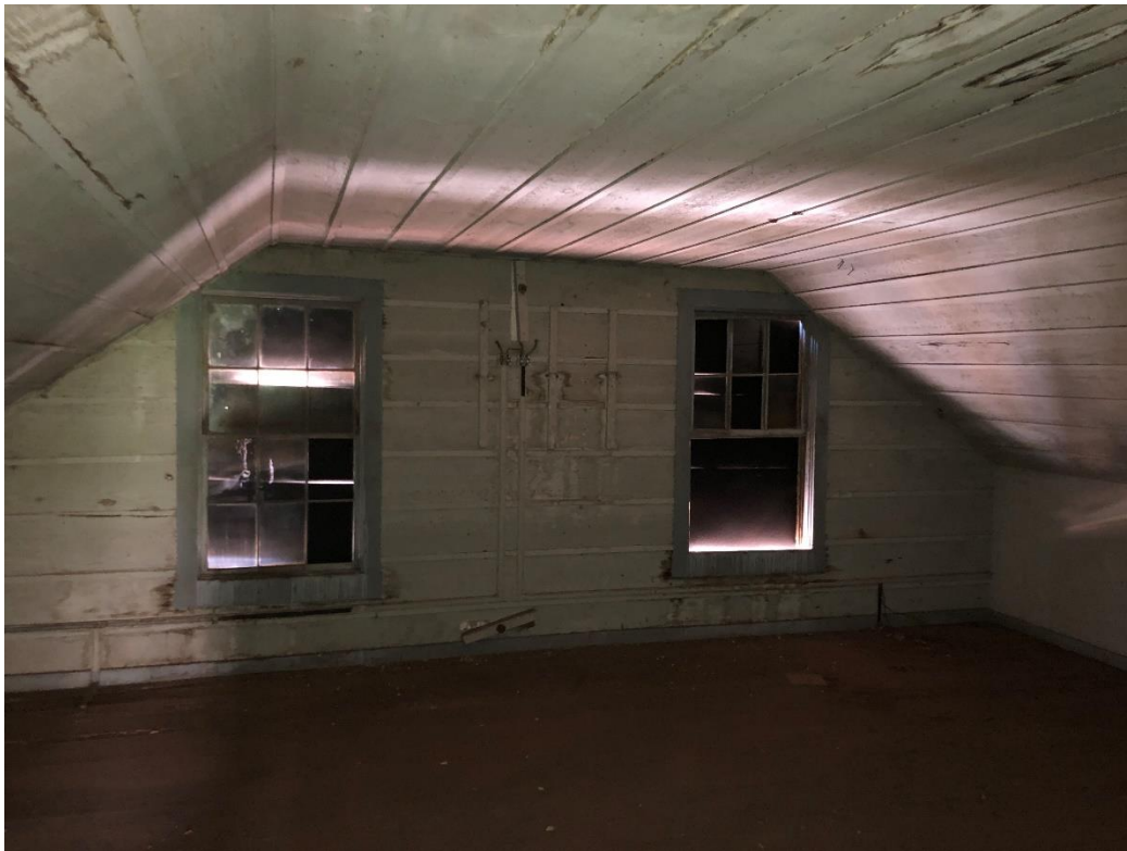
Figure 19: South attic room.
