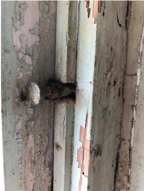
Figure 25: Typical spring sash holder used in all windows except one.
