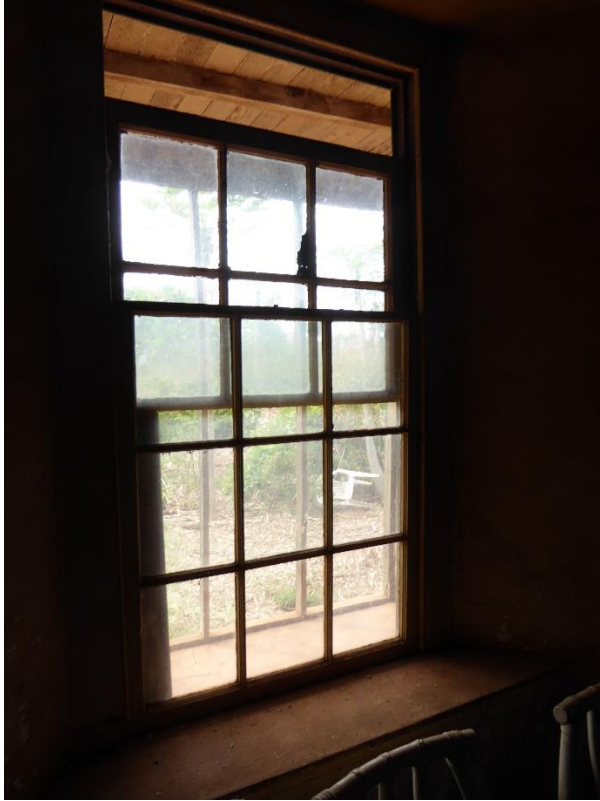
Figure 28: Typical 6 over 9 light window sash.
