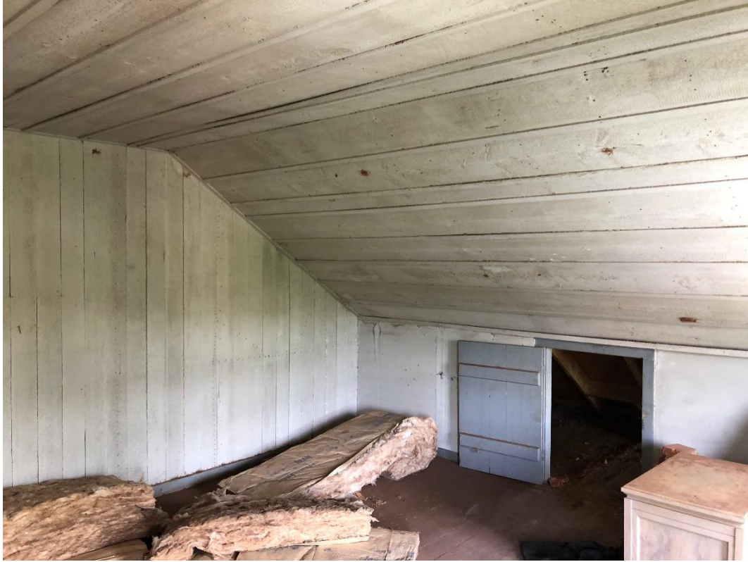
Figure 20: Southwest corner of north attic room
