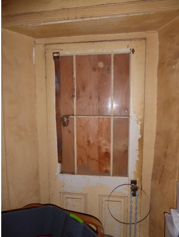
Figure 33: Interior of Door "C". Exterior was boarded up.
