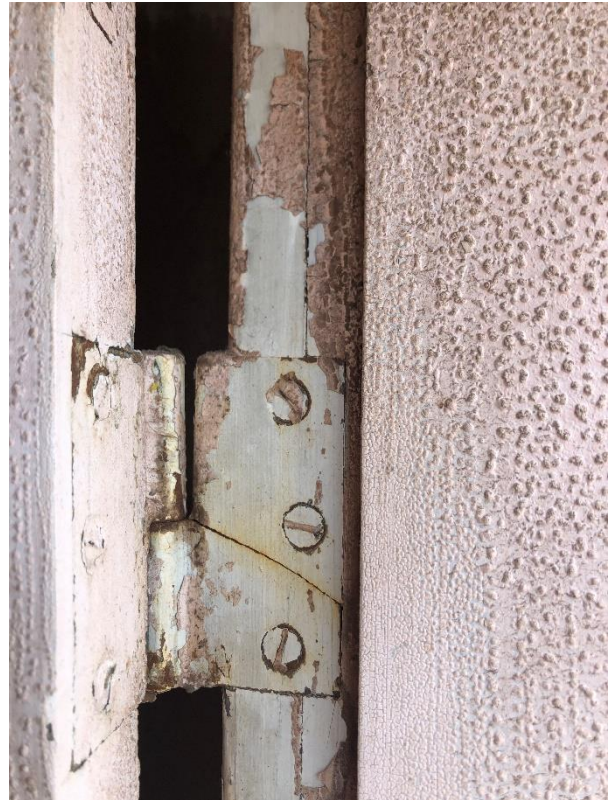
Figure 39: Door U shown on the left. Cracked upper hinge at Door U.
