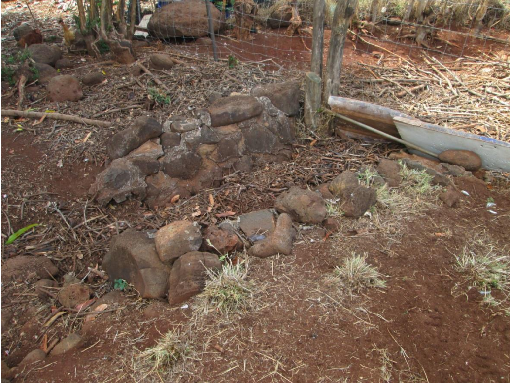
Figure 10: Remains of the foundation of the former structure at north part of the site.
