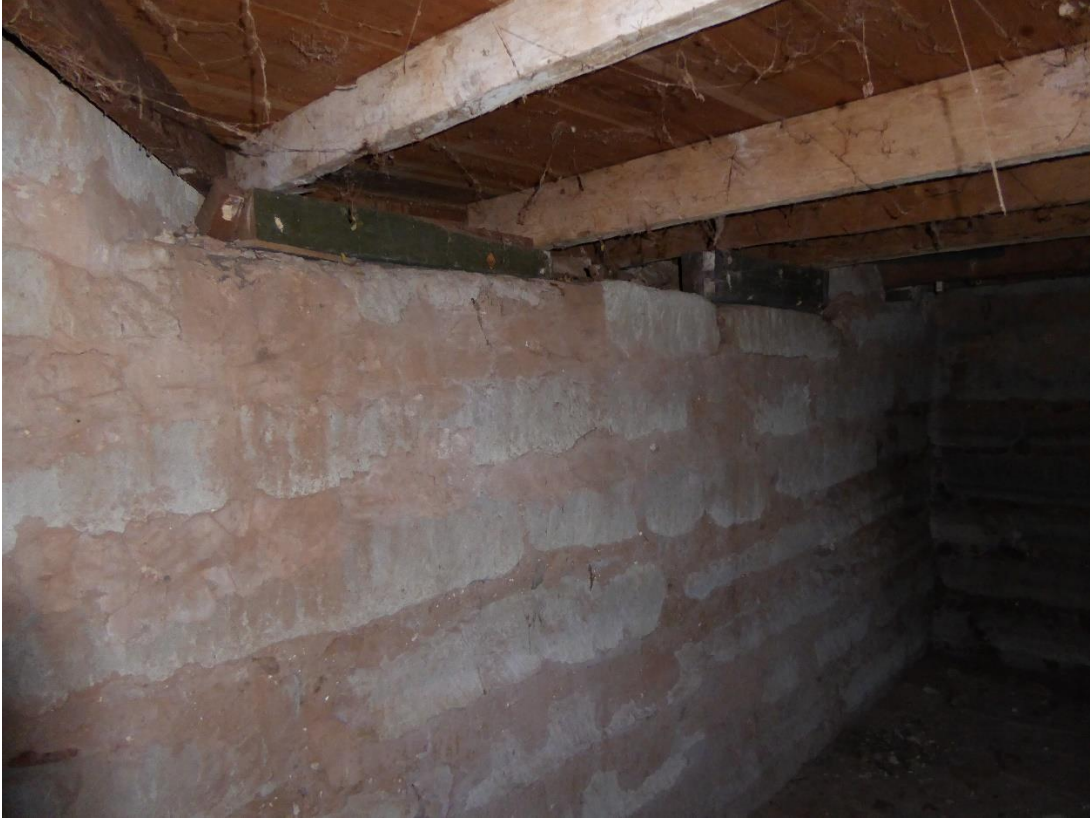
Figure 4: Portion of cellar wall
