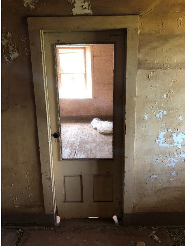
Figure 36: Door Q from hallway (screen door).
