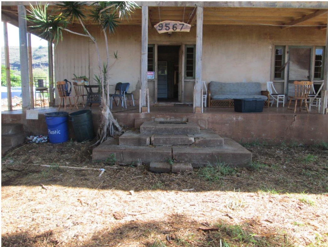
Figure 47: Stair at center of south elevation.
