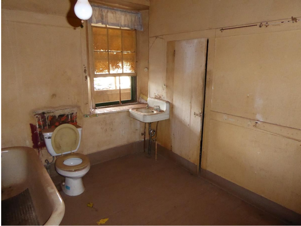
Figure 54: Bathroom showing the sink, storage closet door and window.
