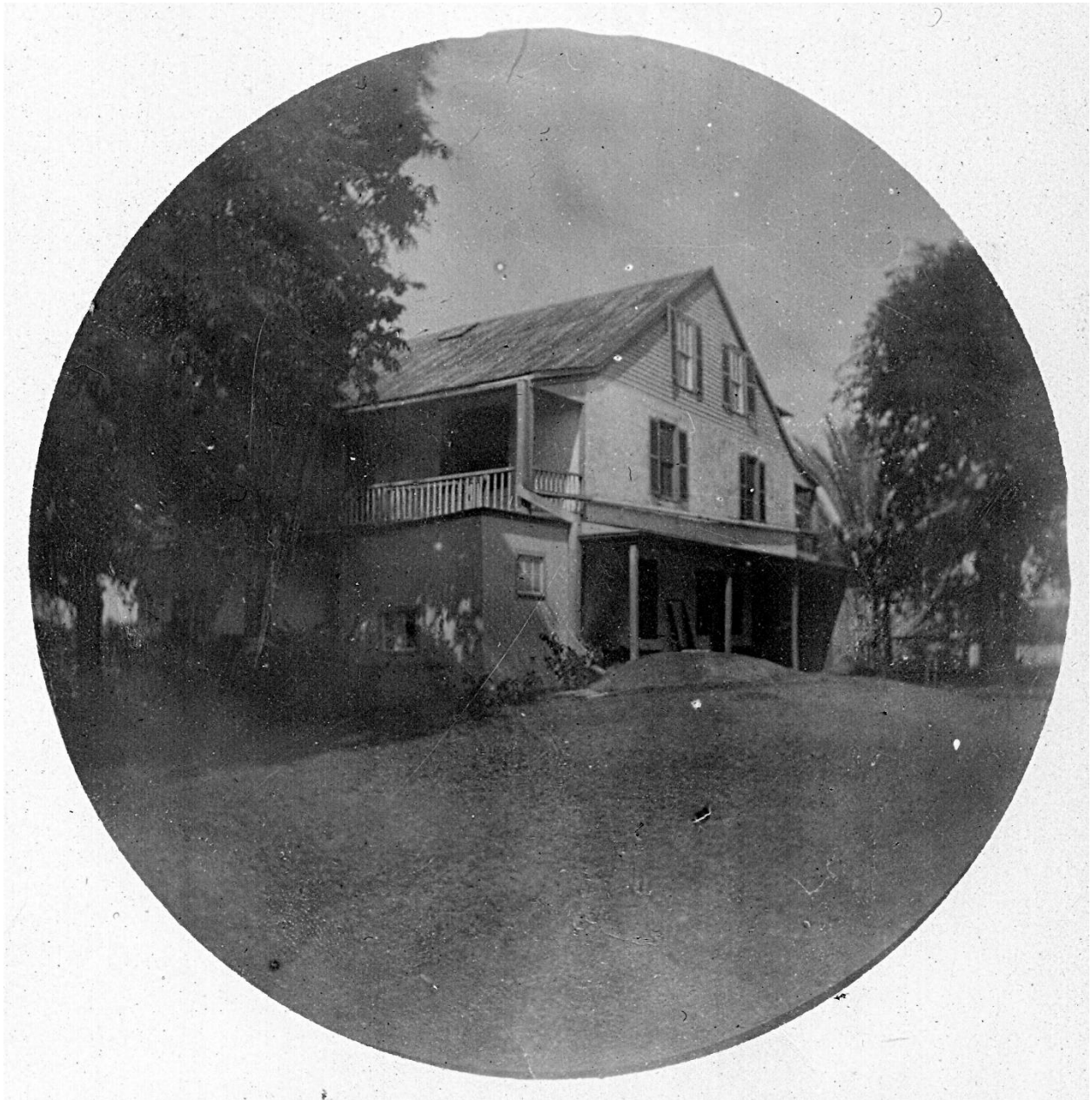
Figure 1: Likely the earliest photo of the house, taken of the northeast corner. Note the gutter and collector system for the cistern.
