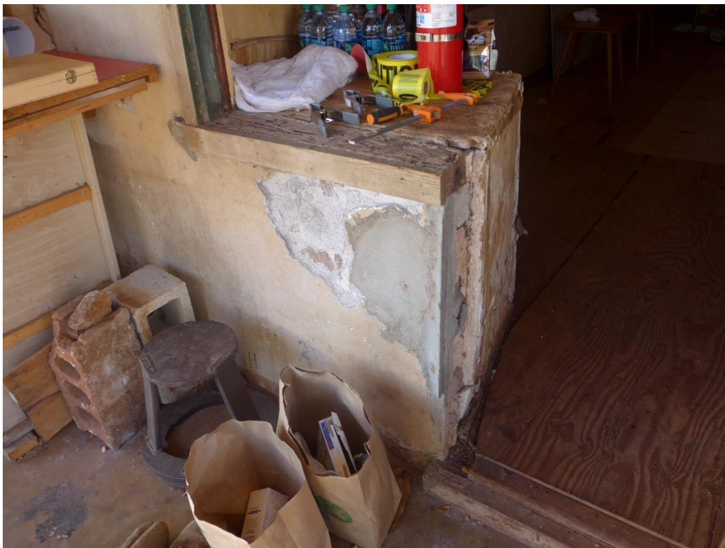
Figure 29: Photo taken in 2015 showing the jamb and sill of the previous window 7.
