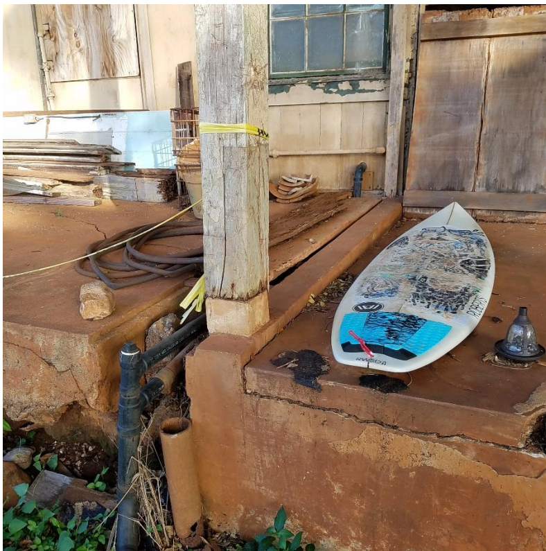
Figure 51: Trench on west side
