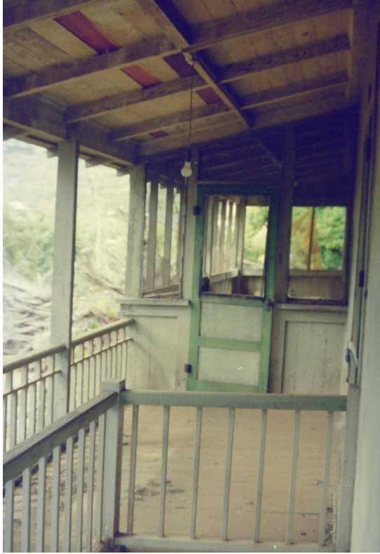
Figure 52: Former screened portion of west upper deck.
