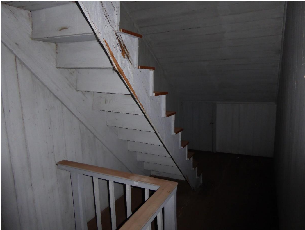
Figure 45: Stair from attic level to former roof hatch.
