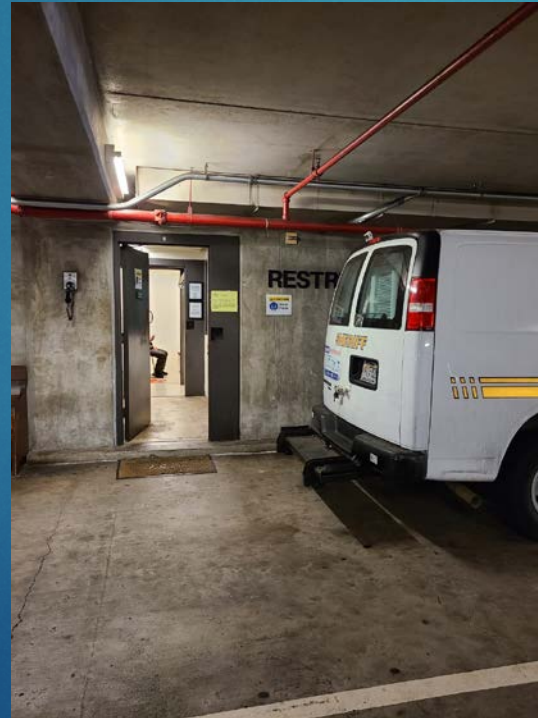
Custodies transfer from van to cell block in open parking structure
