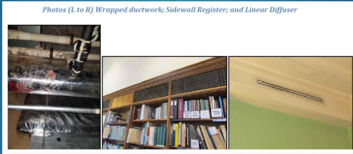
Wrapped duct work; Sidewall register; Linear diffuser
