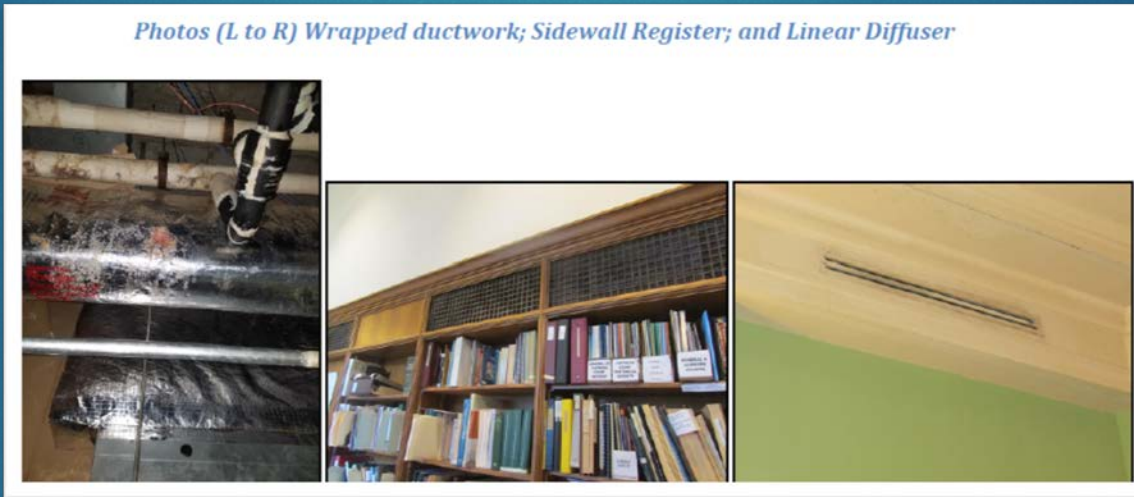
Wrapped duct work; Sidewall register; Linear diffuser
