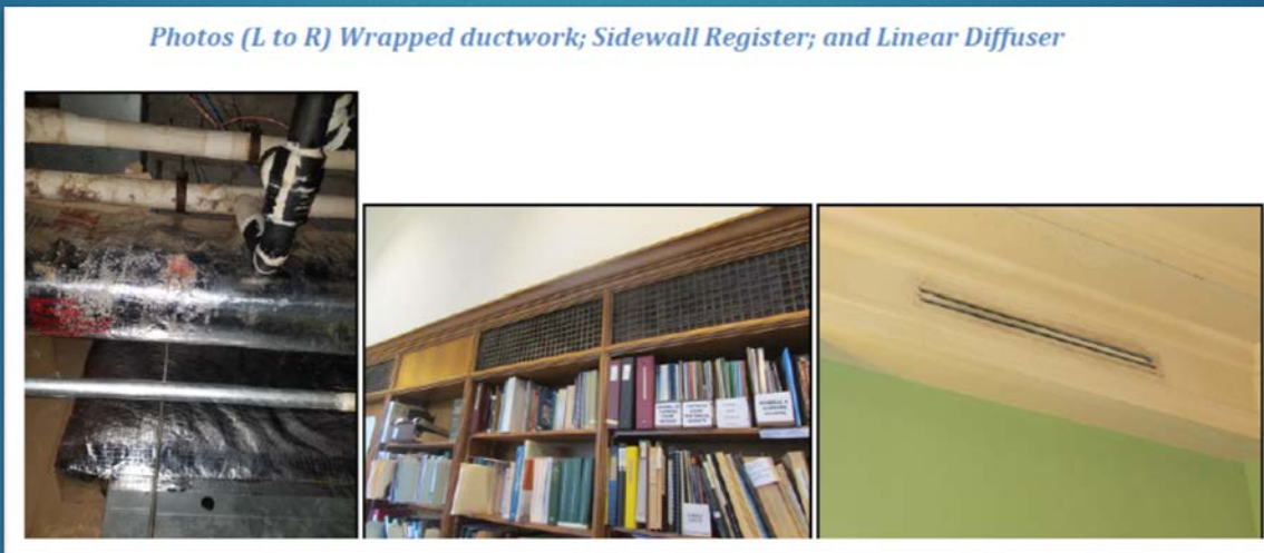
Wrapped duct work; Sidewall register; Linear diffuser
