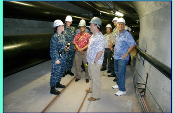
Senator Gabbard checked out the lower tunnel next to the fuel pipe system during a tour of the underground fuel tanks at the Navy's Red Hill Fuel Site on March 5th 2014. From left to right: Lt. Commander Angela Watson, Captain Mark Wheeler, Senator Will Espero, Senator Josh Green, Carlton Saito (Senator Gabbard's Committee Clerk), Gary Gill (Deputy Director of the Department of Health), and Senator Gabbard.
