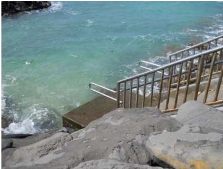
SHORELINE REVETMENT ALLOWS SAFE PUBLIC OCEAN ACCESS
