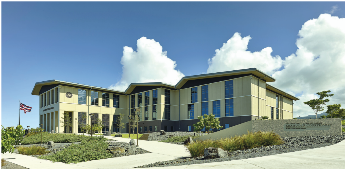
The new Keahuolu Courthouse, Kona, Hawaii island, September 2019. Photo courtesy of AHL and Andrea Brizzi Photography.
