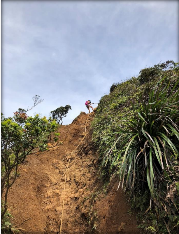
This shows a user created alignment with too steep of a grade, resulting in tread failure
