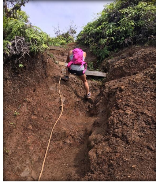
Deferred maintenance leading to design failure
