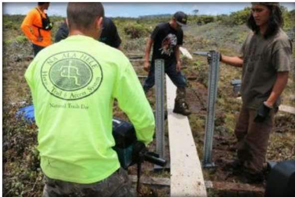
Na Ala Hele Staff constructing the Alaka‘i Swamp Boardwalk
