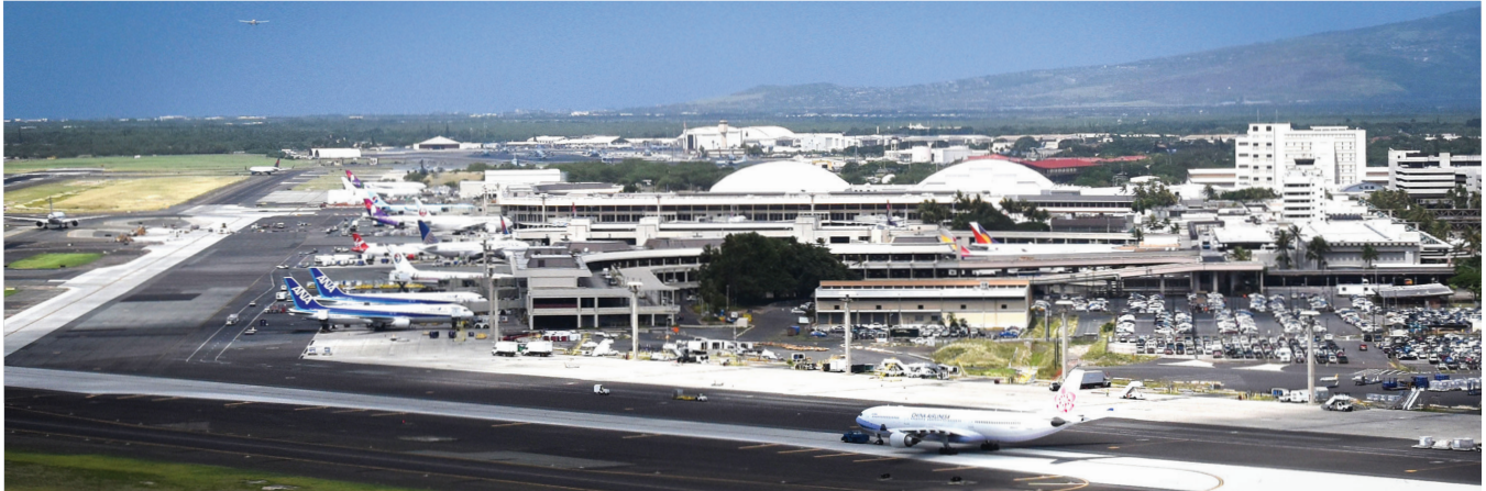
PHOTO: HAWAII DOT AIRPORTS DIVISION
