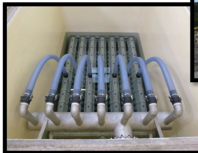
▲ New treatment building ◀ Microfiltration basin
