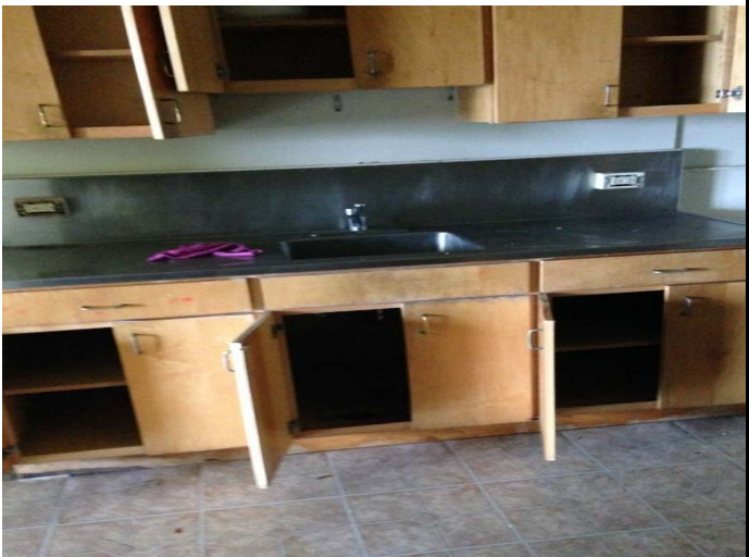
Before: Typical unit prior to renovation.
