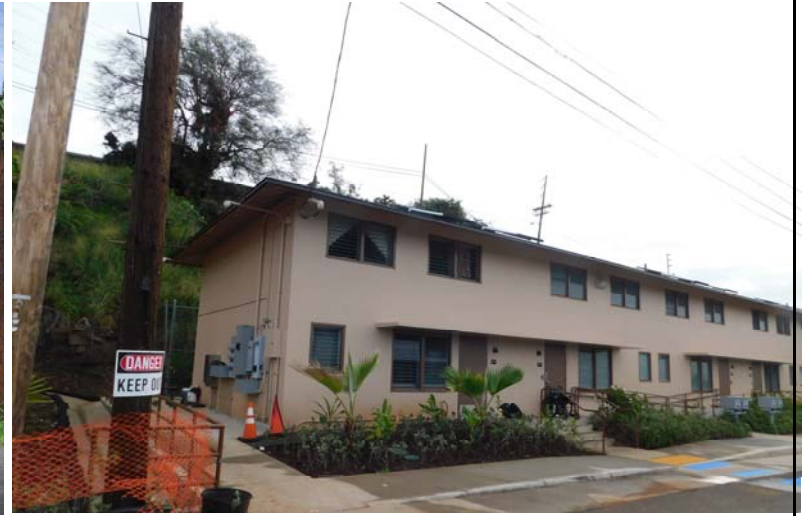
After: ADA sitework upgrades.
