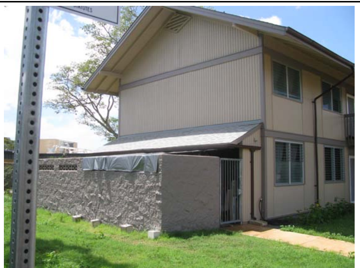
After: Typical post renovation building
