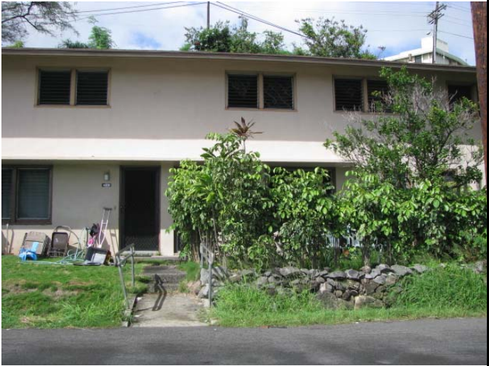
Before: Unit entrance prior to ADA upgrades.
