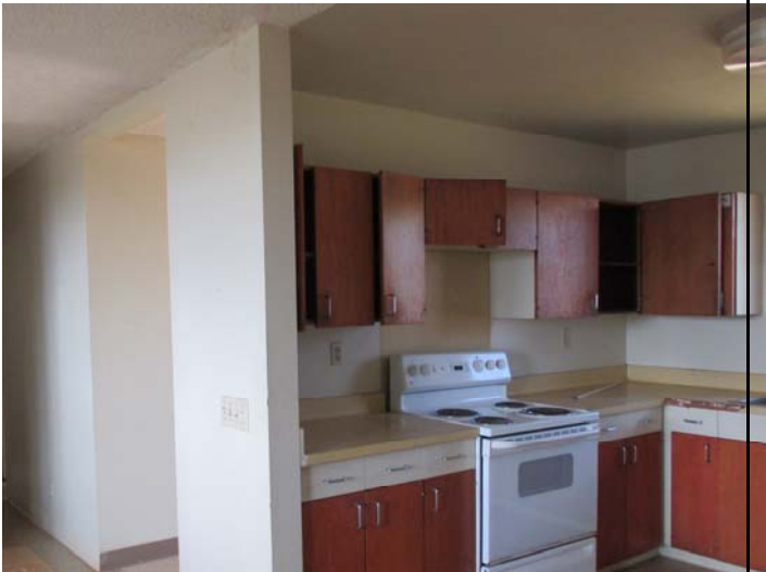
Before: Typical pre-renovation unit
