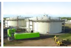
Renewable Natural Gas (Honouliuli WWTP)
