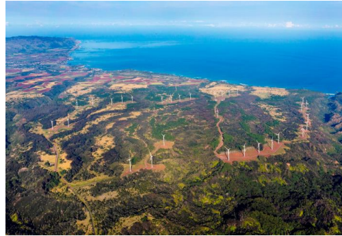
Kawailoa Wind Power, O'ahu
