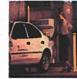
1998 Hawaiian Electric helps install the state's first electric vehicle "rapid charging station."
